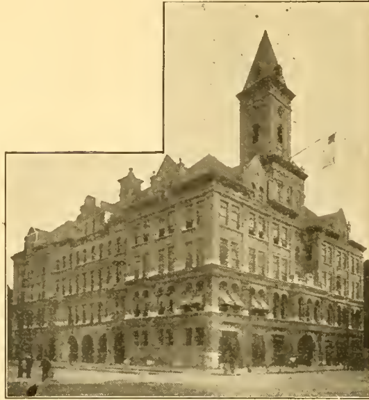
CITY HALL BUILDING, BIRMINGHAM
