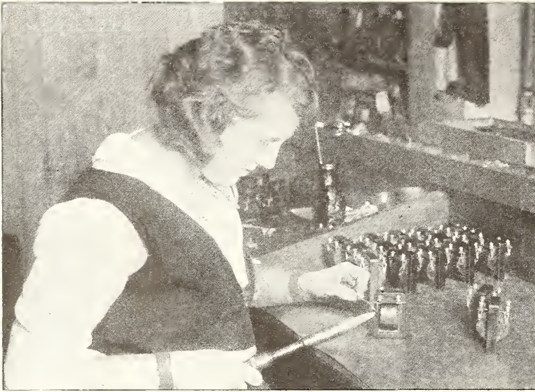
SOLDERING TRANSFORMER LEADS—A DELICATE JOB
