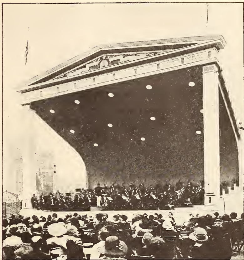
THE NEW STAND BUILT FOR THE N. Y. PHILHARMONIC ORCHESTRA Willem Von Hoogstratem is shown conducting his orchestra of 106 men, at one of the Stadium concerts in New York. The stand, erected by the General Electric Company, is portable and adapted especially for the broadcasting of the orchestra's programs. The two black dots, one above the other, to the right of the left-hand pillar, are the microphones
