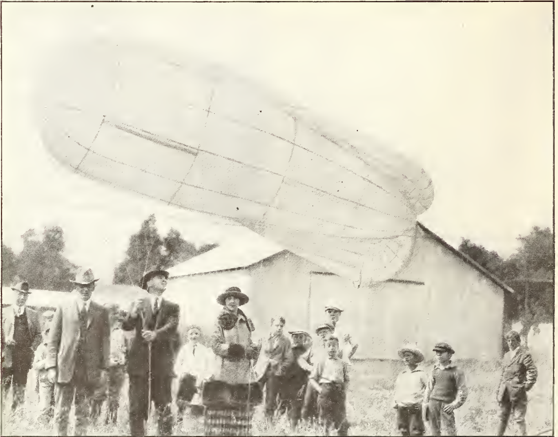
USING A YOUNG BLIMP TO SUSPEND THE ANTENNA
