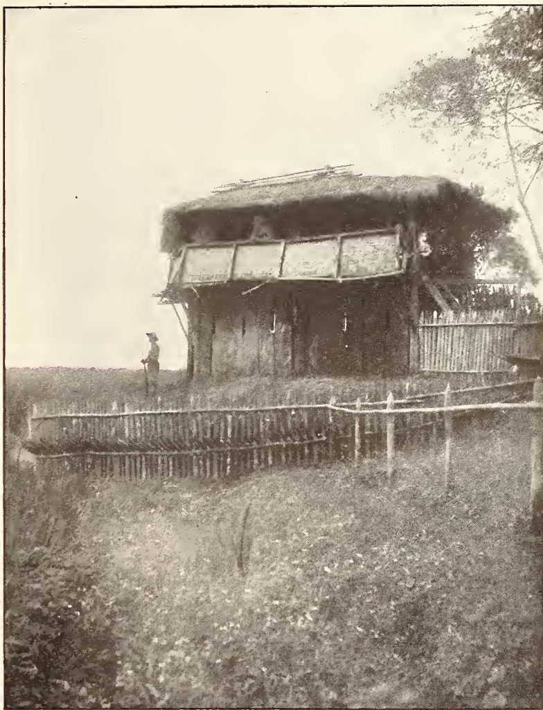
A CORNER OF THE DEFENSES OF KON TUM Showing the stockade with its sharp-pointed posts, set like bayonets against a possible attack by man or beast
