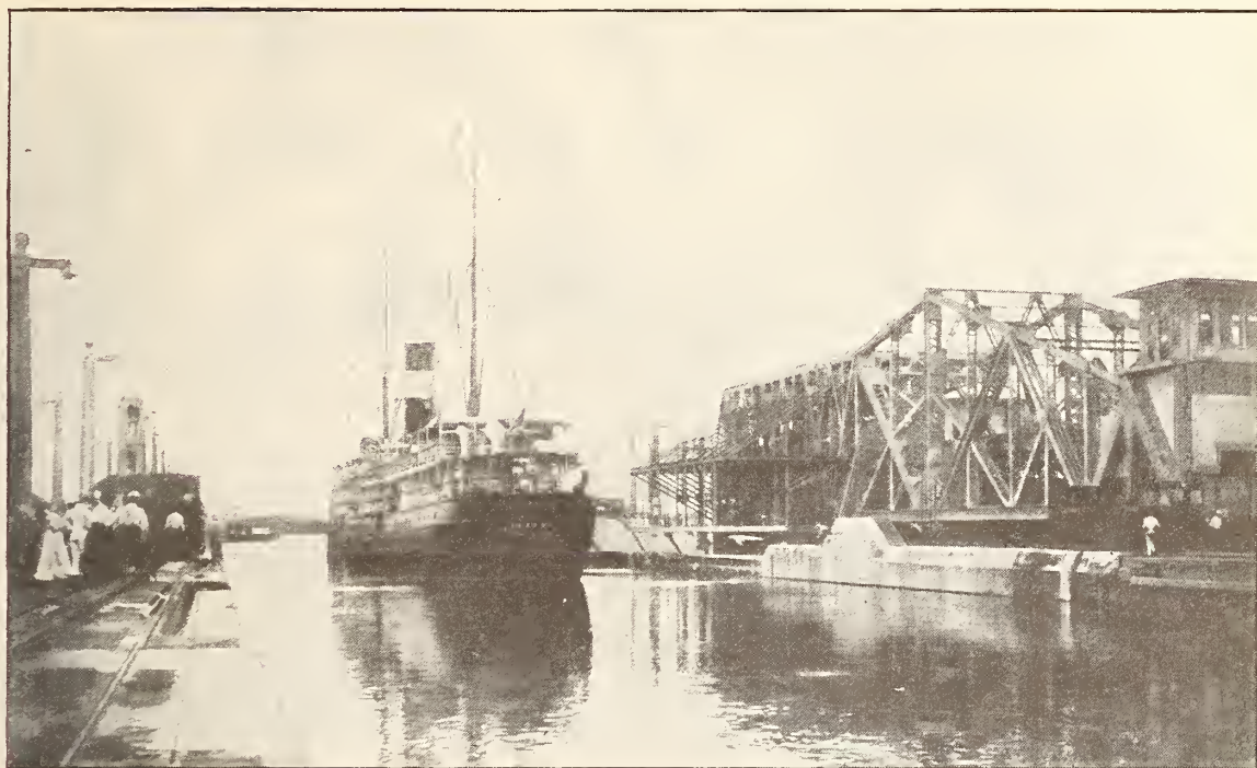
THE ALLIANCA—FIRST LINER TO GO THROUGH THE GATUN LOCKS
