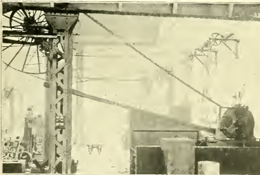
TYPE "C" MOTOR OPERATING MACHINE TOOLS.
