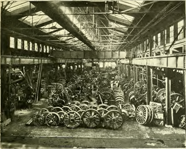
WHEEL LATHE SHOP; BALDWIN LOCOMOTIVE WORKS.
