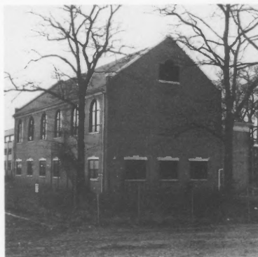
This older building houses the gymnasium and swimming pool.
