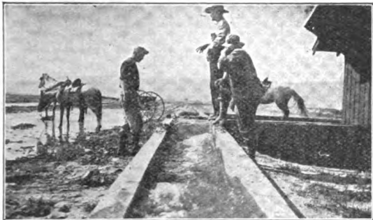
This pumping plant irrigates 160 acres
