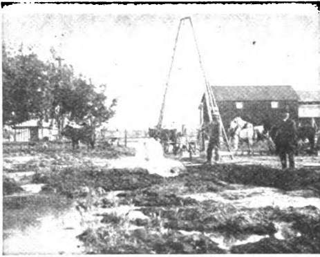
TYPICAL ARTESIAN WELL IN MADERA COUNTY
