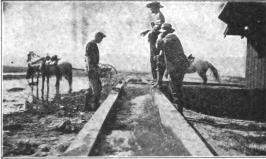
This pumping plant irrigates 160 acres
