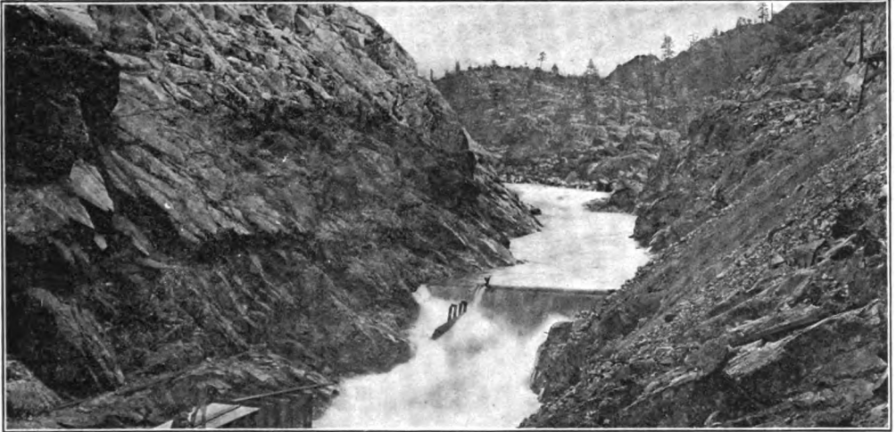
It was November. Tomorrow the first concrete would be poured if . . . . By nine that evening it was raining. By morning, the boom of the river filled the canyon and before daylight faded into early night the flood had smashed the flume, run away with the wreckage and the river, leaping joyously over the trembling dam, was back in its old bed
