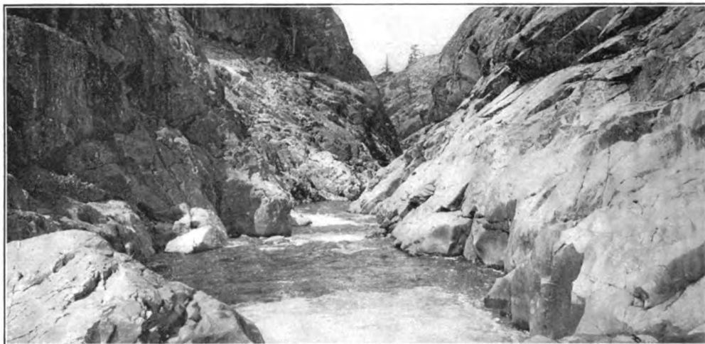
In the rocky canyon of the South Yuba, just below where the river leaves Lake Spaulding, a spot was selected as the site for the titanic dam. It was imperative that the foundations of the dam be finished by fall, before winter, with its twenty feet of snow, swooped out of the sky. Millions were at stake in this race with the snows of the Sierra
