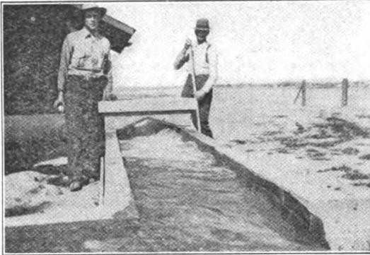
200 inches of pure water raised 25 feet
