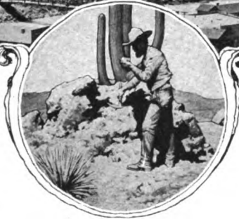
The rich copper district of northern Sonora, sending its concentrates to the smelters, is directly tributary to the wealth of Arizona
