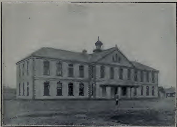
The New Printing Press Building, Chentu, China.
