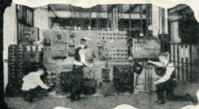
Students Working on Massive A. C. Control Equipment
