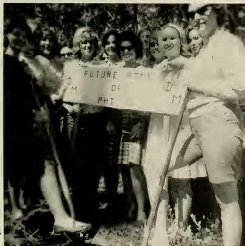
We really are good carpenters.
