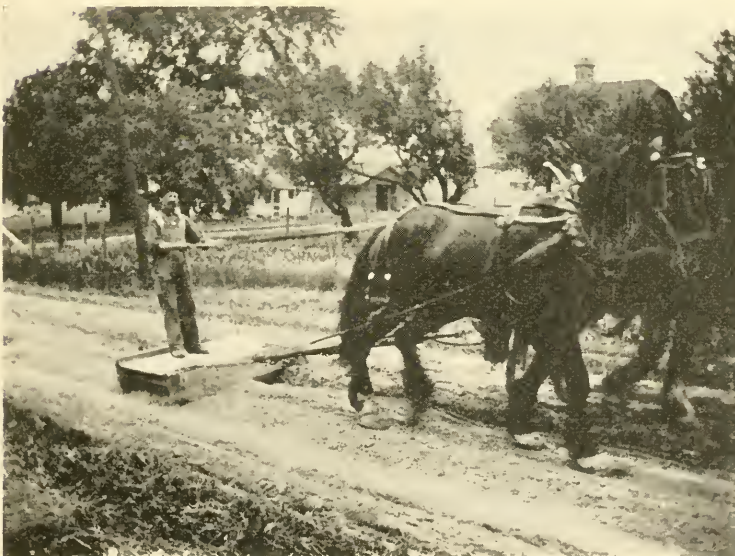
Fig. 40. King Road Drag in Use.
