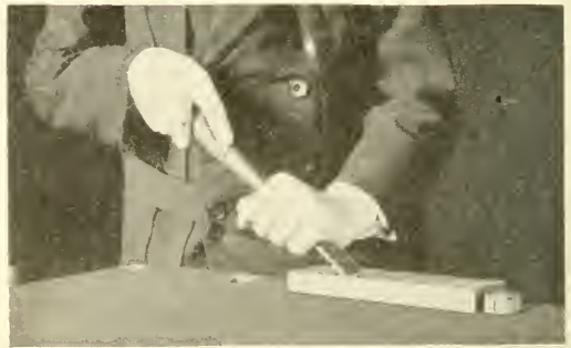
Fig. 22. Whetting the Beveled Side of a Chisel.
