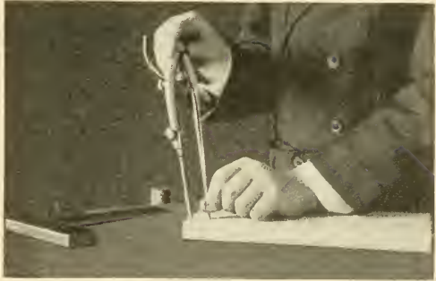
Fig. 7. Swinging an Arc with a Compass.
