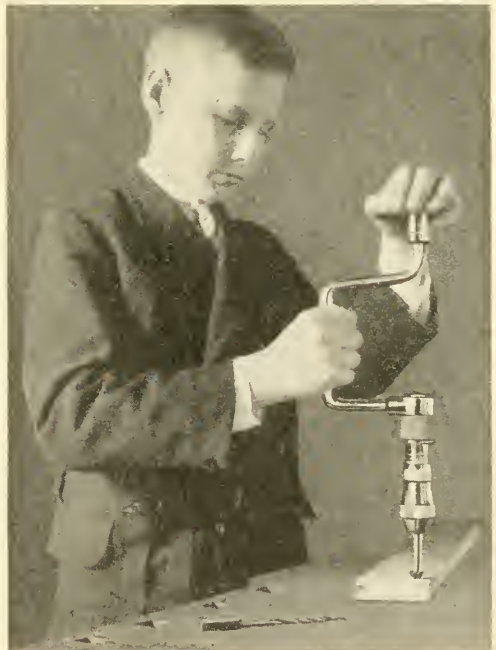
Fig. 13. Countersinking a Hole.
