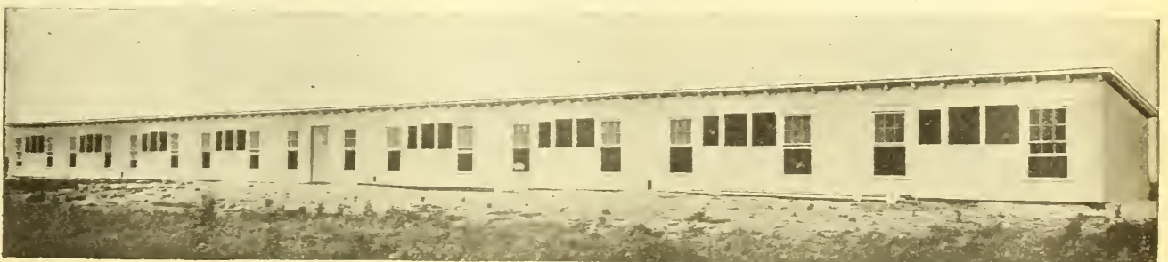
Fig. III.—Curtain-front house in which experiments were conducted at the West Virginia Station.
