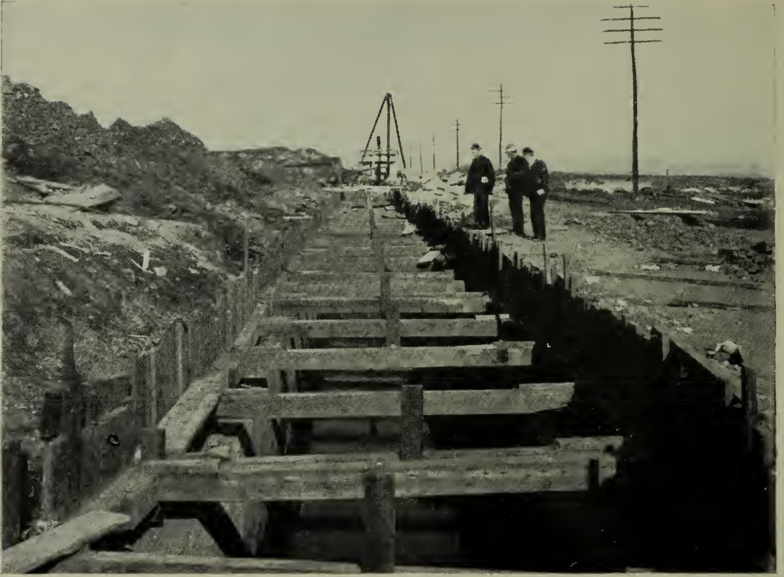
VIEWS—STORM DRAIN OUTLET, MIDDLESEX AVENUE, 10 FEET X 7.5 FEET.
