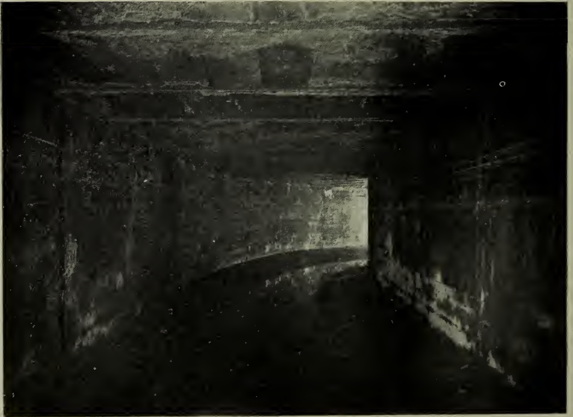
VIEWS—STORM DRAIN OUTLET, MIDDLESEX AVENUE, 10 FEET X 7.5 FEET.
