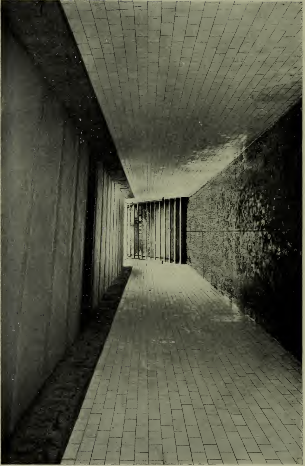
THORNDIKE-STREET SUBWAY, WEST SOMERVILLE.
