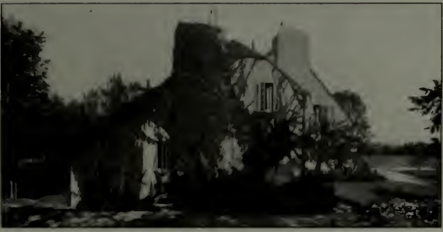
The gable end which houses laundry and storeroom is as pleasing as the garden side.
