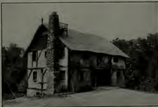
Structural timbers are frankly recognized as timbers, not as geometrically sawed pieces of wood. Unfortunately the chief charm of this garage, its color, cannot be reproduced
