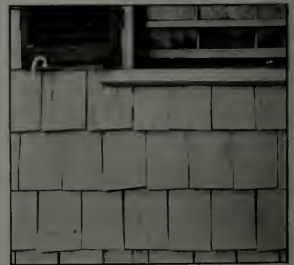
An enduring white stain has supplanted the whitewash used in an earlier day, giving the desirable intense whiteness of lime and, like lime, making the shingles lie flat.
