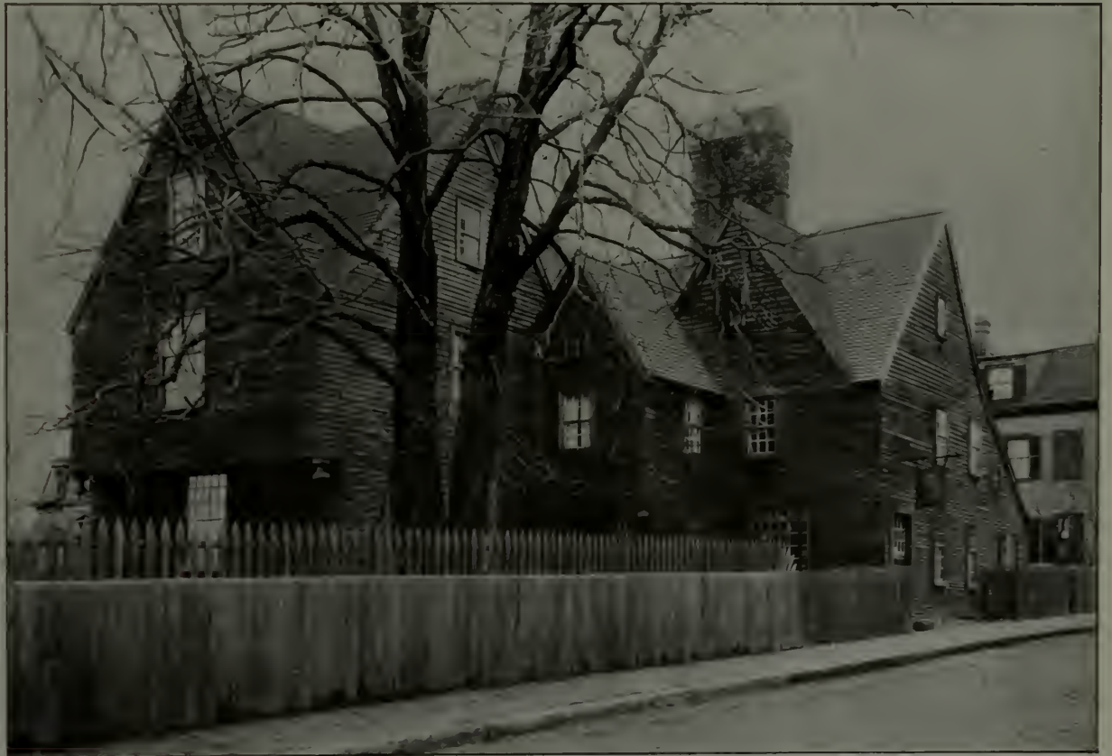
The original of Hawthorne's "House of the Seven Gables" shows a number of Gothic characteristics, such as the steep roof, the massive chimneys, and the second-story overhang with its carved "drops"
