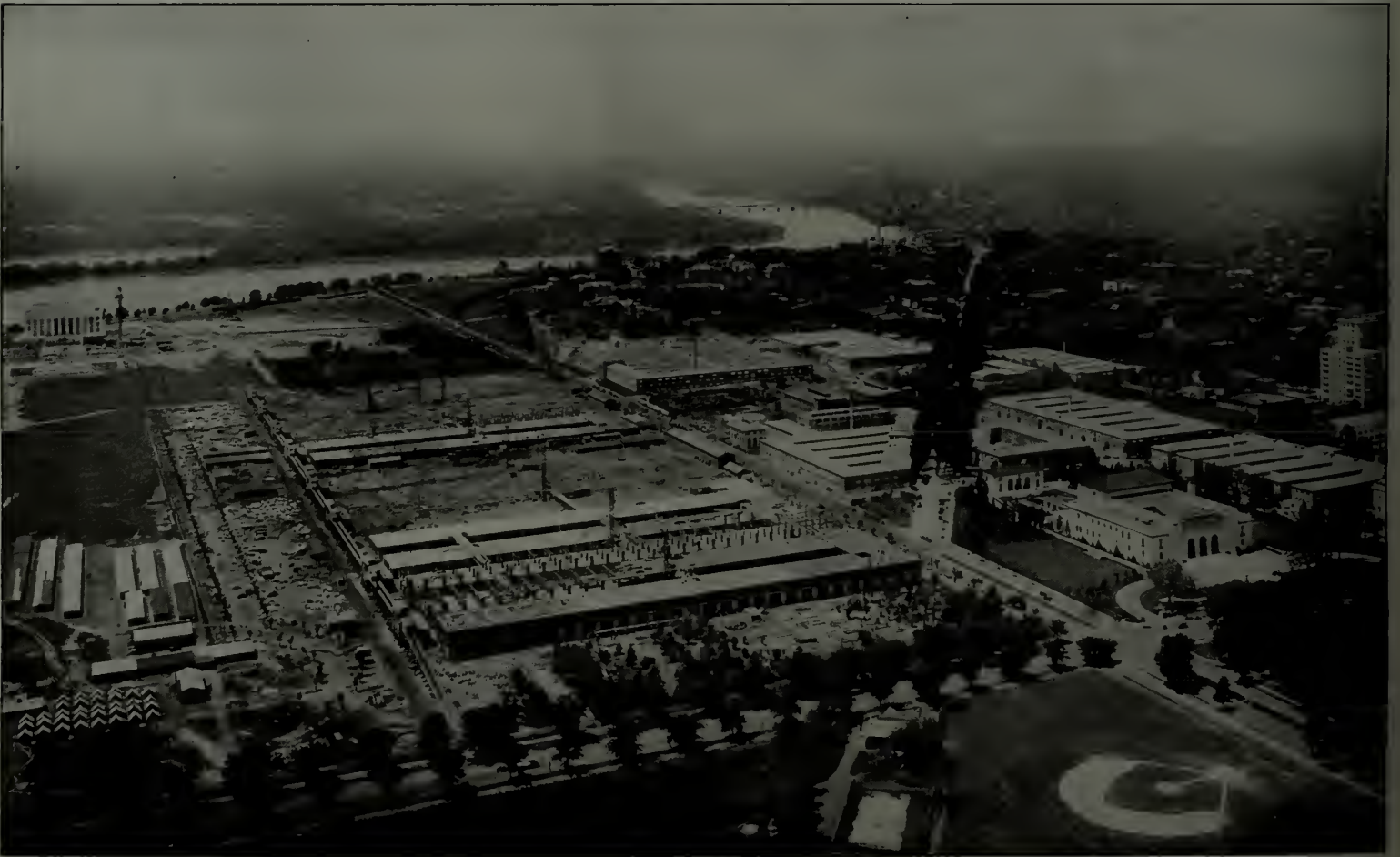
View showing temporary Government building operations west of Seventeenth Street, and between the Lincoln Memorial and the Pan-American Union building. The vista from the Washington Monument to the Lincoln Memorial is being preserved. The buildings on Government ground are to be razed after the war
