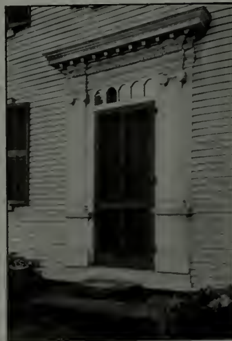
Although paint has preserved the clean-cut wood details of the old Stebbins house doorways, time has noticeably rounded the edges of the stone doorsteps.
