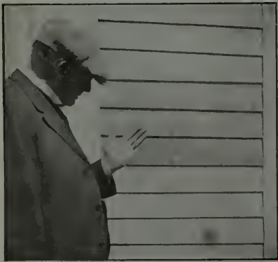
When the ingredients in paint are wrong it chinks off, the result of saponification and consequent washing off of the oil, leaving the white pigment, which gives no protection.
