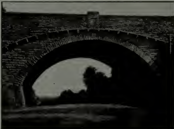
A good possibility ruined by the machine symmetry, the network of tuck pointing, and the knife-edge straight line at the top
