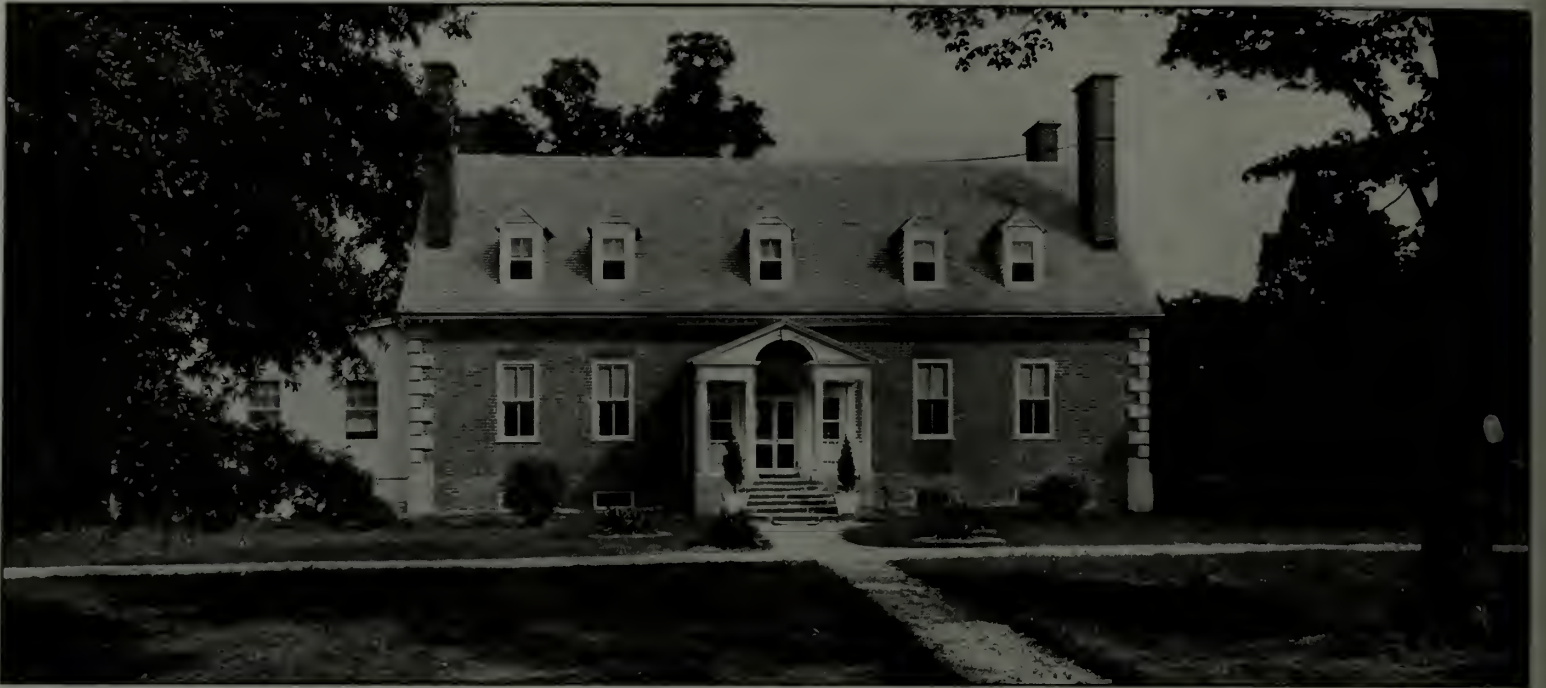
Historic Gunston Hall, the Colonial home of Washington's friend, George Mason, which has been relieved of its questionable "improvements," and stands forth once more in its original simplicity and beauty. It is now owned by Mr. Lewis Hertle
