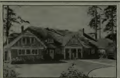
Stained with Cabot's Creosote Stains, C. H. Bebb and C. F. Gould, Architects, Seattle
