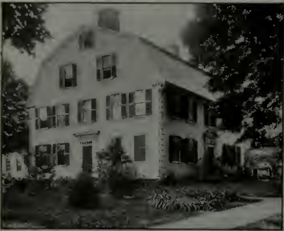
The famous old Stebbins house at Deerfield, built in the eighteenth century, is a monument to the efficiency of paint as a means of preservation.
