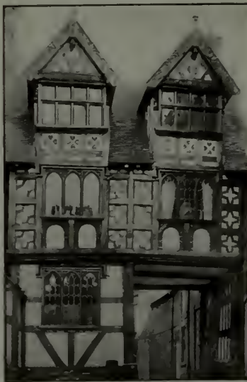
A piece of old and good work spoiled by recent additions in the shape of stenciled patterns masquerading as timbers in the second-story panels, and simulated beams painted on the ground floor wall.
