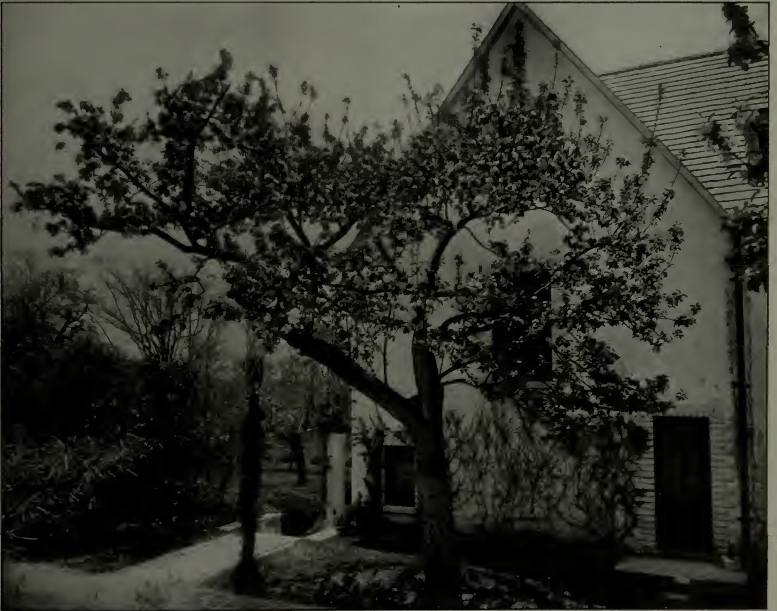
The door in this picture gives on to a landing in the stairs and affords access to the second floor without going through the main part of the house. The apple tree casts welcome shade in summer on the path to the front door and on the side door, and for a week in spring literally forces its blossoms through the window on the stairs
