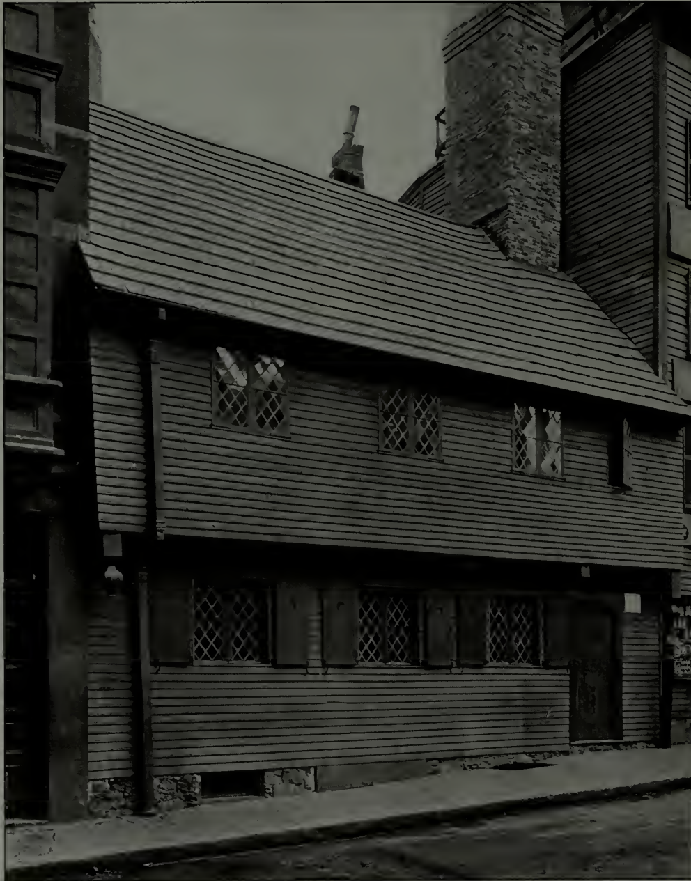
The old Paul Revere house in Boston shows Gothic influence in its casement windows and second-story overhang
