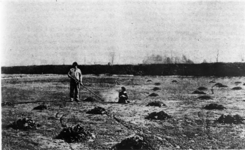
FIG. 3.—BED NO. 12; RAKING OFF SLUDGE DEPOSIT. (MORE DEPOSIT THAN USUAL.)
