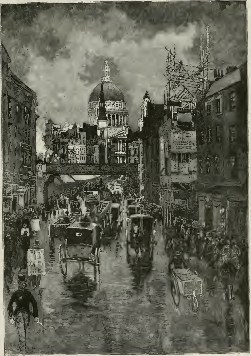
THE WEST FRONT OF ST. PAUL'S, FROM FLEET STREET.
