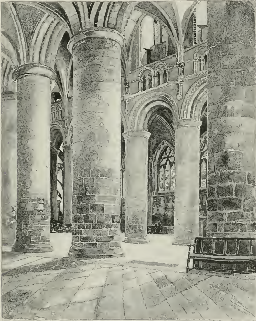
THE NAVE, FROM THE NORTH AISLE.
