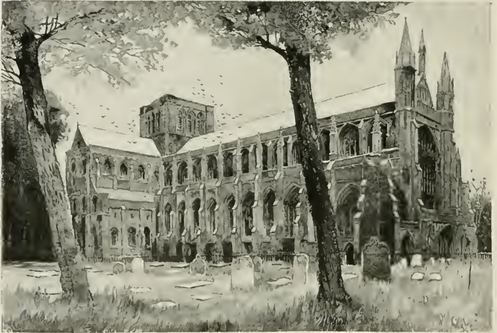
THE NAVE AND TRANSEPT, FROM THE NORTHWEST.
