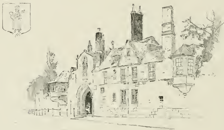
NORTHEAST GATEWAY TO THE CLOSE.
