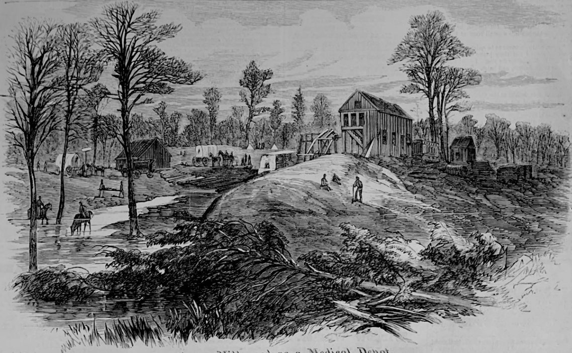
Steam-Mill used as a Medical Depot.
