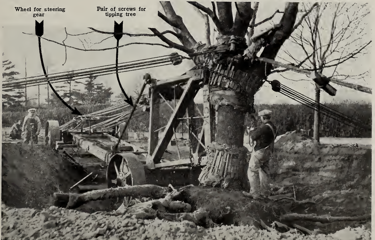
Our steel tree-mover No. 20, designed for large deciduous trees. With this we can move trees 70 feet high, 50 feet wide, with an area of roots 45 feet in diameter. There are two screws used to swing the tree over. The cradle is padded, to distribute the pressure. The rear wheels are steered by a wheel, enabling trees 80 feet high to get around sharp corners.
