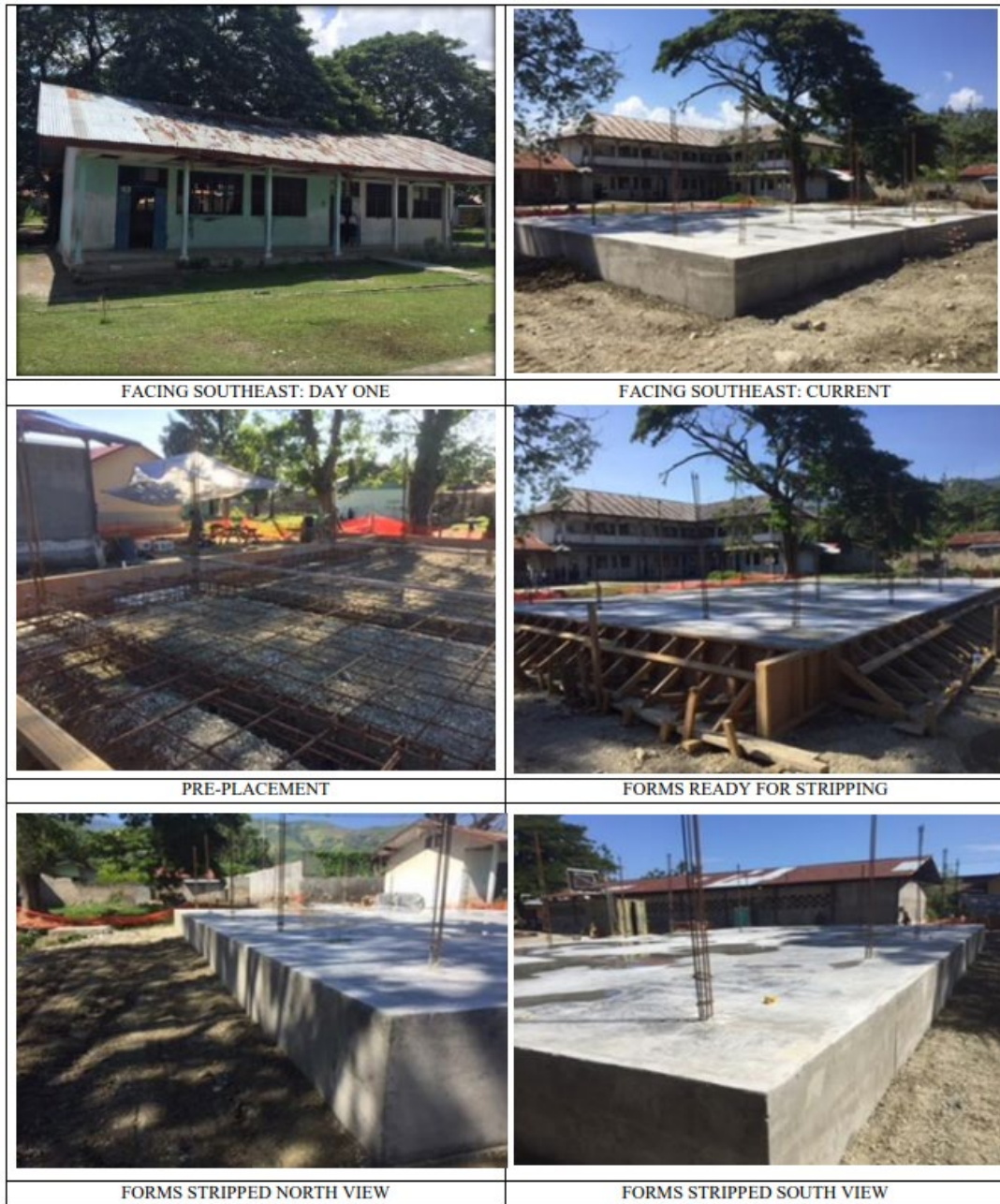
Figure 8 School Building Renovation (Source: Project Report from the 30 th NCR)
