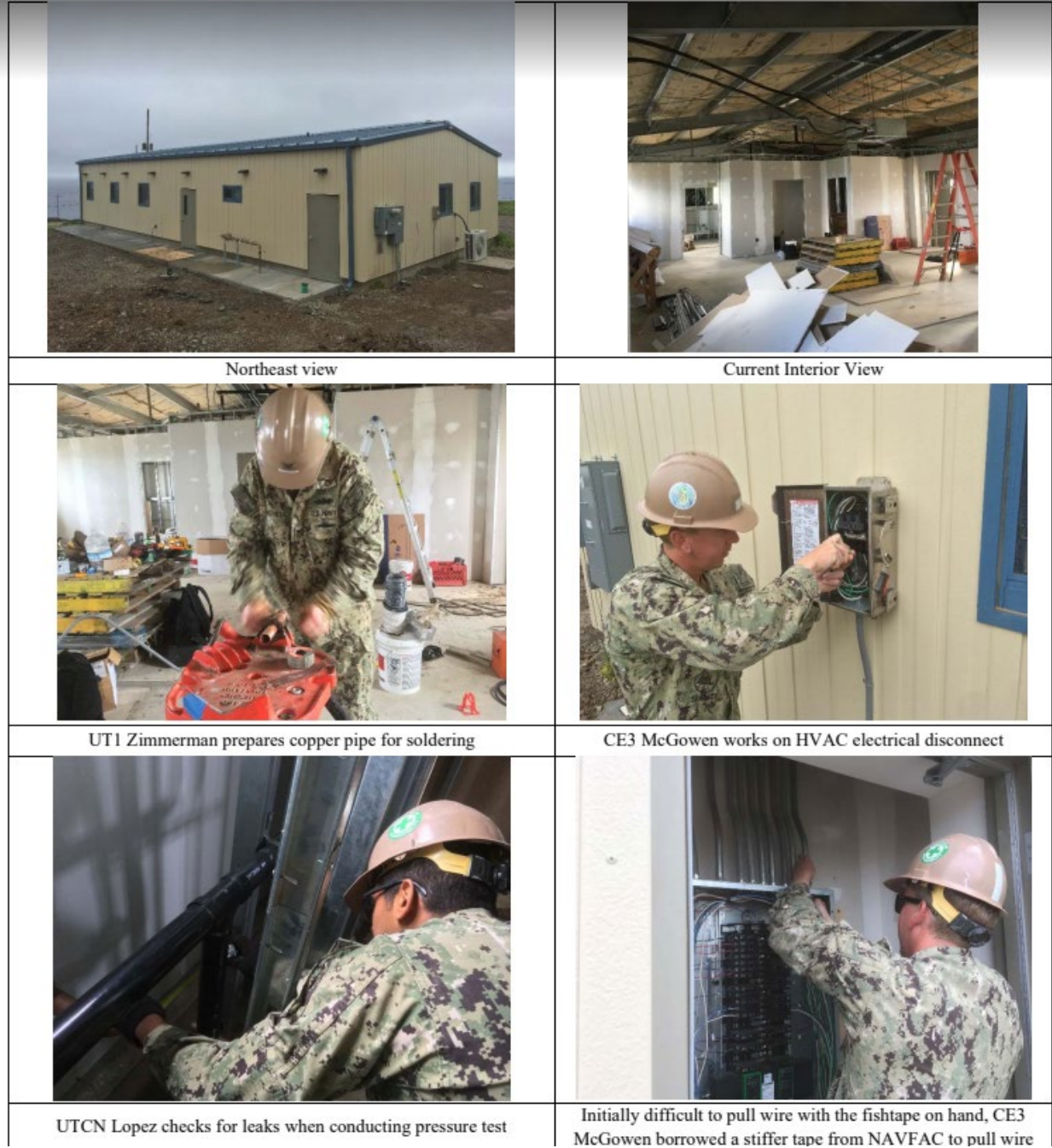
Figure 6 30' X 60' pre-engineered building construction (Source: Project Report from the 30 th NCR)
