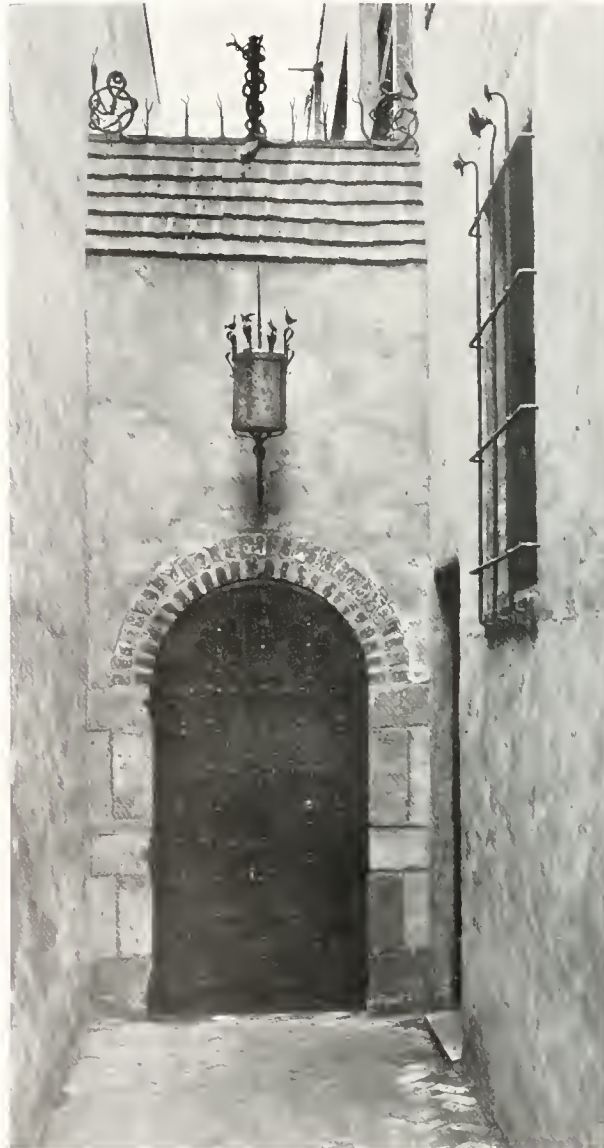
LANTERN AND OTHER IRONWORK OF SAMUEL YELLIN'S STUDIO-SHOP
