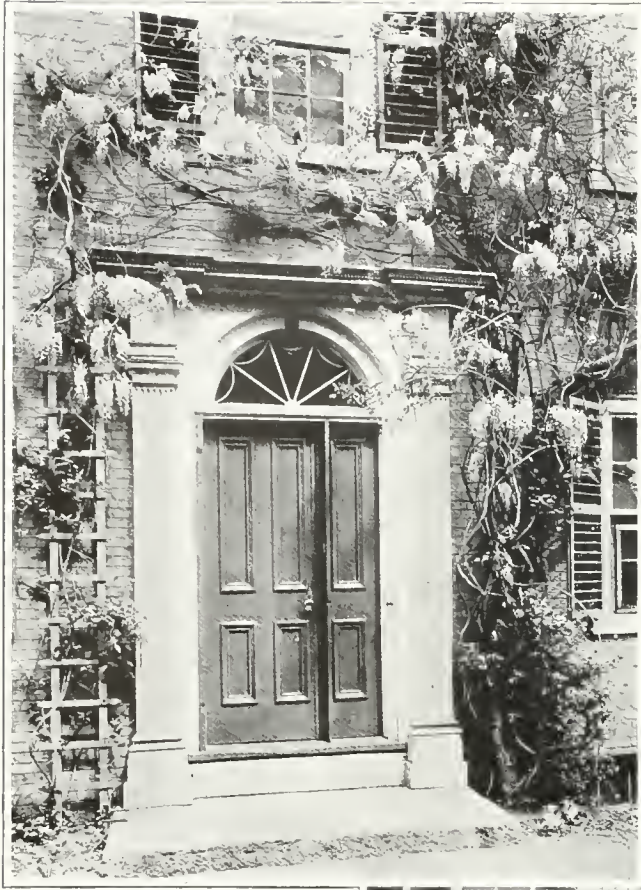
AN OLD COLONIAL DOORWAY FRAMED WITH WISTARIA
