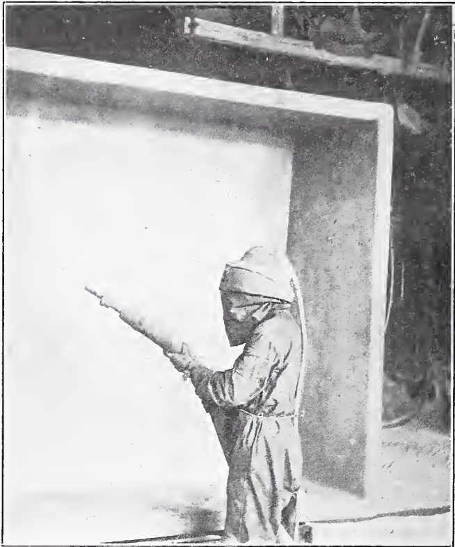
FIG. 4.—Sandblasting a rectangular tank.
