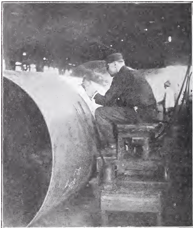
FIG. 2.—Oxyacetylene welding.
