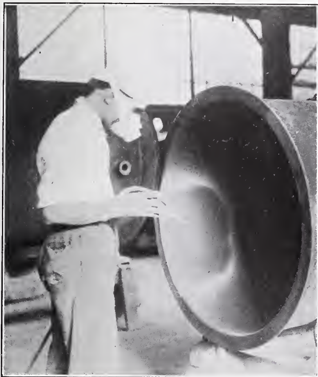
FIG. 5.—Spraying a steel tank.
