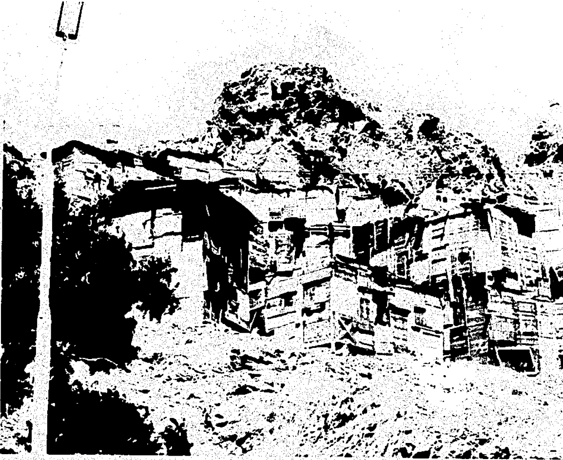
FIGURE 8. Typical housing in one of Aden's shanty districts. These dwellings constitute severe fire and health hazards. Densities of 5 to 6 persons per room are not uncommon. (U/OU)
