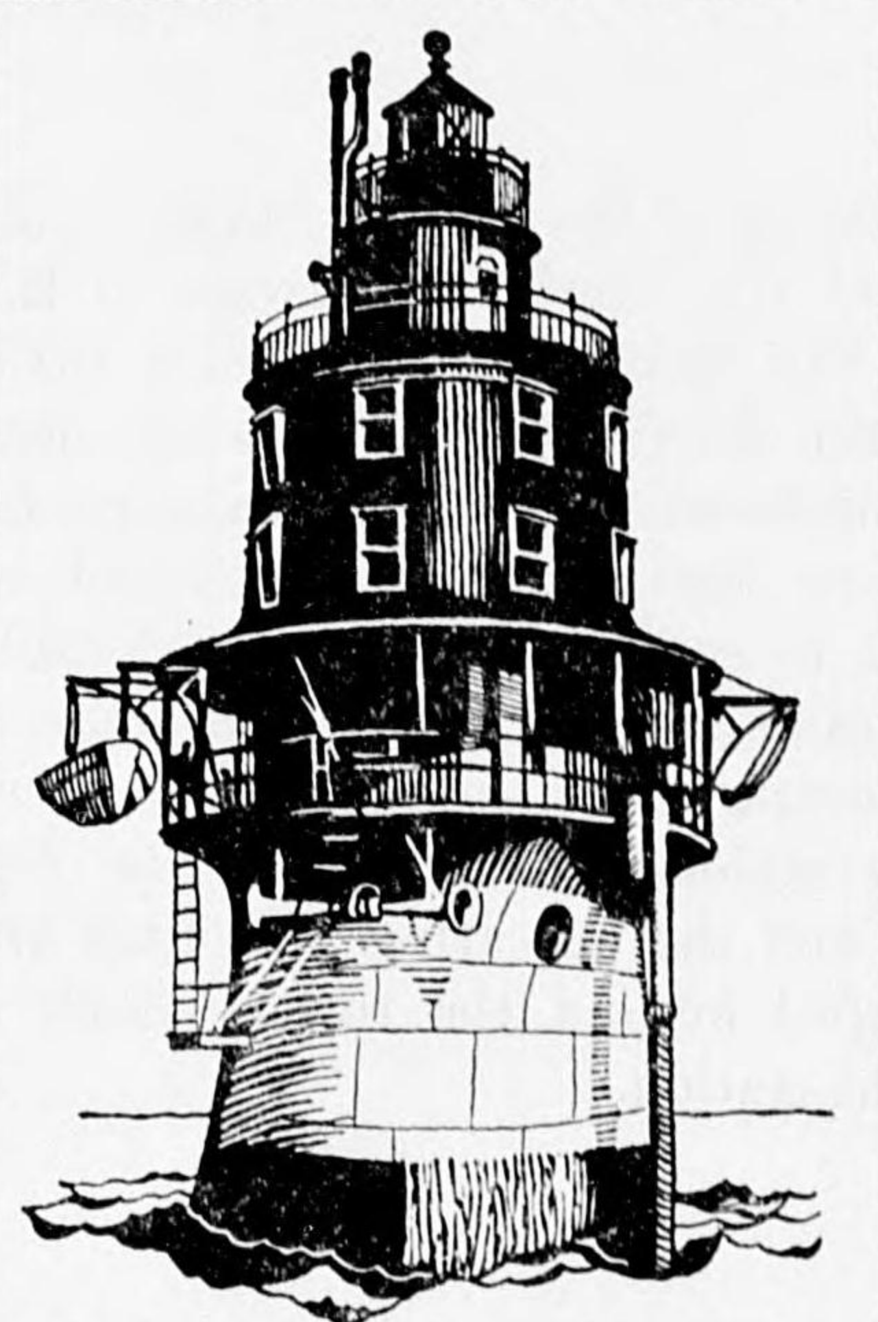
CYLINDRICAL CAISSON STRUCTURE
