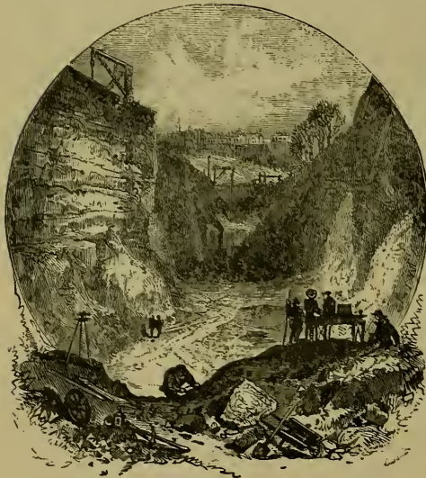
ENTRANCE TO BALTIMORE TUNNEL.
