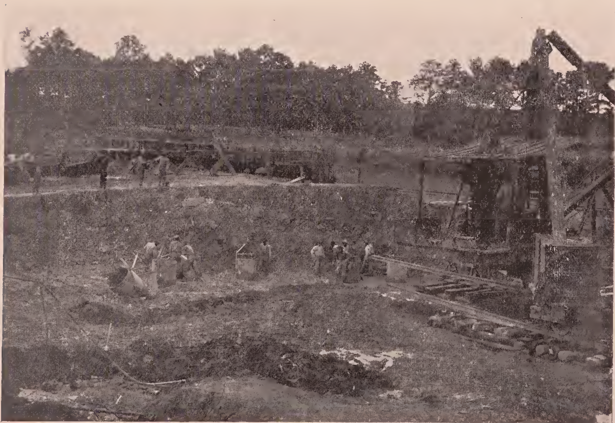
FIG. 2.—PIT OF WASHINGTON HYDRAULIC-PRESS BRICK COMPANY, HARMAN, ANNE ARUNDEL COUNTY.
