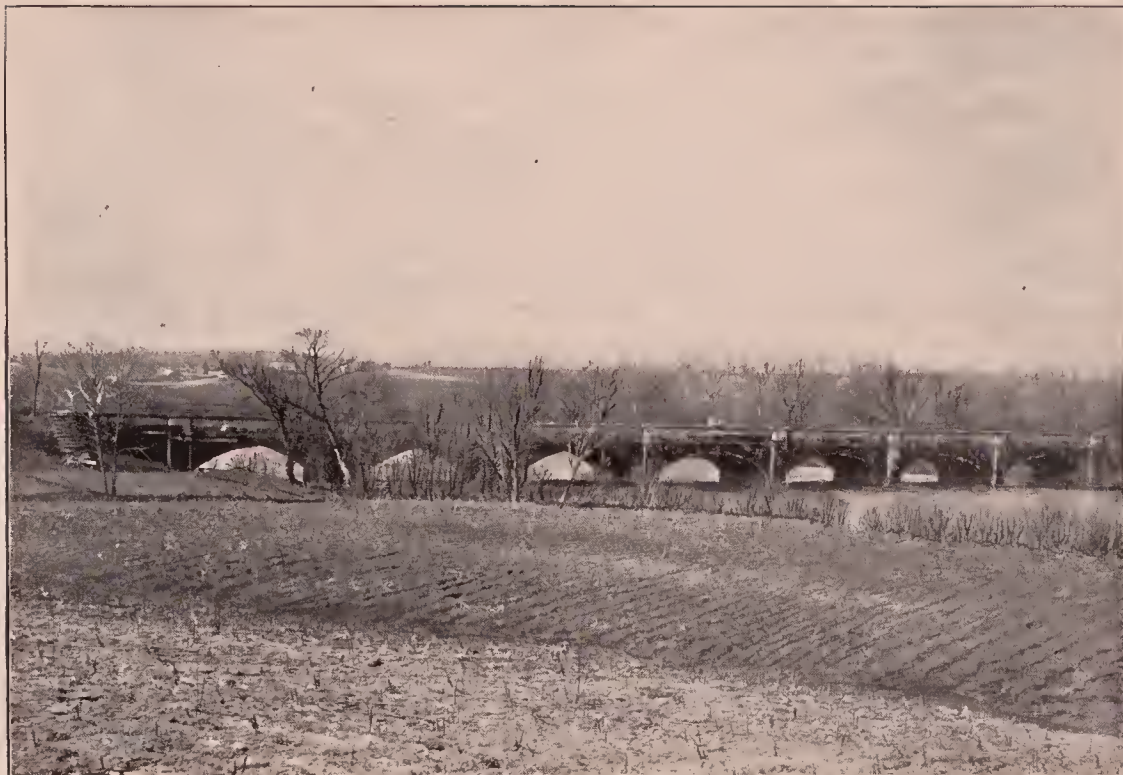
FIG. 1.—VALLEY FARM-LANDS OF THE PIEDMONT PLATEAU, WITH MONOCACY AQUEDUCT, FREDERICK COUNTY.
