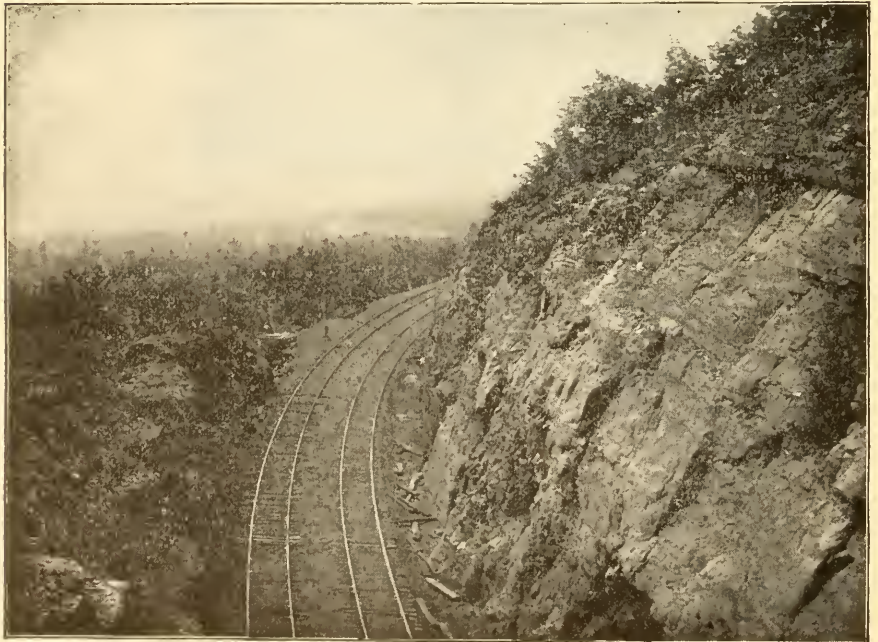
NORTHERN APPROACH TO PARADISE TUNNEL.
