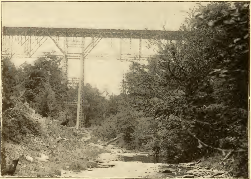
MILL CREEK BRIDGE, (118 FT.) DANSVILLE, N. Y.
