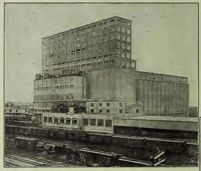
PHOTO shows the 3,800,000 bushel Terminal Grain Elevator of the B. S O. Railroad Company at Baltimore, Md., in which 9½ miles of Diamond Grain Belts, weighing 149 tons, were installed during the early part of 1925. This is one of the fastest grain handling plants in the world.
