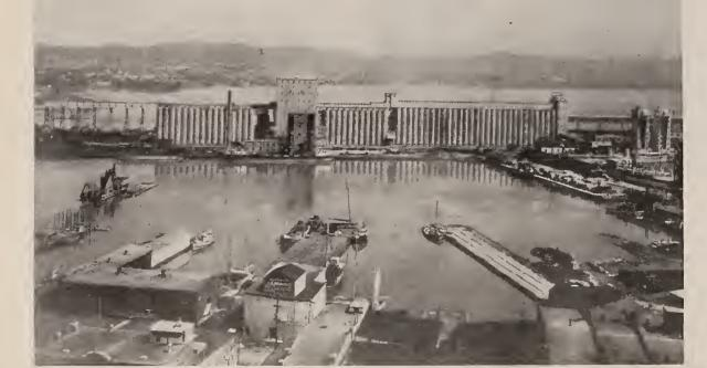
SHOWING 2,000,000-BUSHEL ADDITION AND NEW MARINE TOWERS OF QUEBEC ELEVATORS
