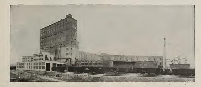
Santa Fe Elevator A in Kansas City operated by the Davis-Noland-Merrill Grain Co. ranks among the world's largest elevators, having an unloading capacity of 200 cars and a loading capacity of 250 cars within a normal working day. Its total storage is 6,000,000 bushels.
