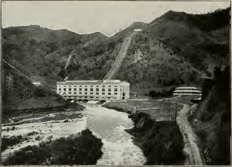
HYDRO-ELECTRIC PLANT, LAGES. PENSTOCK AND VALUE HOUSE ABOVE; CLUB HOUSE OF OPERATORS BELOW
