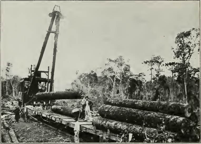
THE "SOUTHERN BRAZIL LUMBER AND COLONIZATION COMPANY" LOADING PINE LOGS AT TRES BARRAS, PARANA
