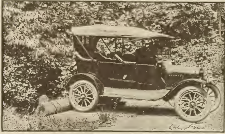
This is a "turn-around" on a narrow road that runs alongside a steep bank in Roland Park, Maryland. It consists of a heavy log laid flat on the ground, well spiked to two other logs driven into the ground.
