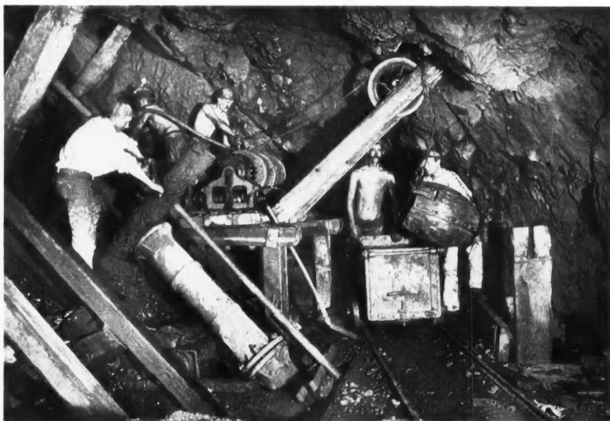
17. ENGINE SHAFT AT THE 406, COOK'S KITCHEN MINE.
