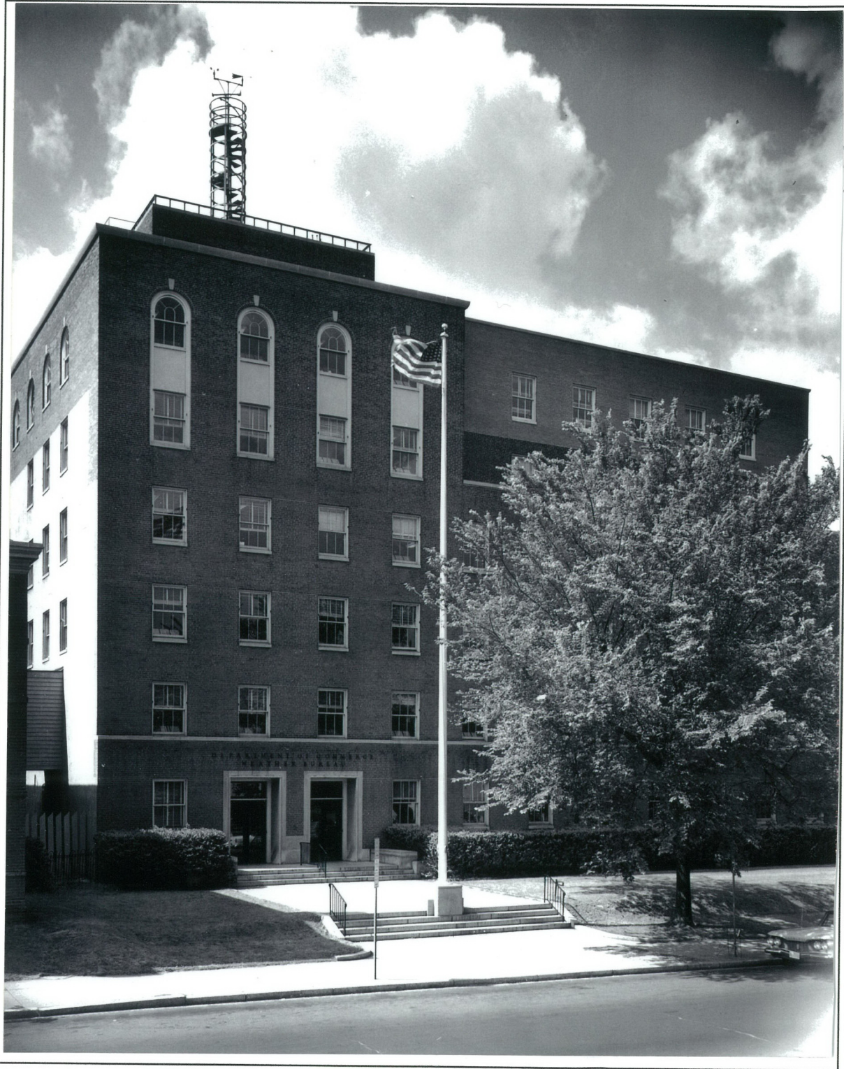
The building at 2400 M Street that was the home of Weather Bureau Headquarters from 1941 until it moved to Silver Spring, Maryland, in 1966. It was built in front of the Ferguson Building that was used as the headquarters for approximately 53 years. The Ferguson Building still existed and was also used, along with the "Old Annex." The top, sixth, floor to the right was not added until 1961.
