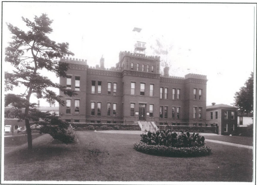
Another view of the Ferguson Building showing a building on the west, similar to that on the east and south (not visible).
