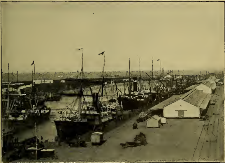
One of the basins in the Buenos Aires docks.
