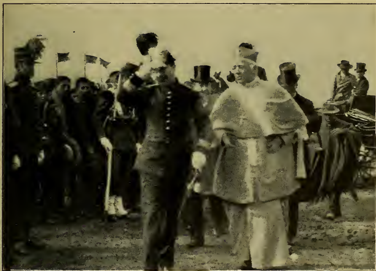
President Montes and the Archbishop just after turning the first shovelful of earth on the new railway.
