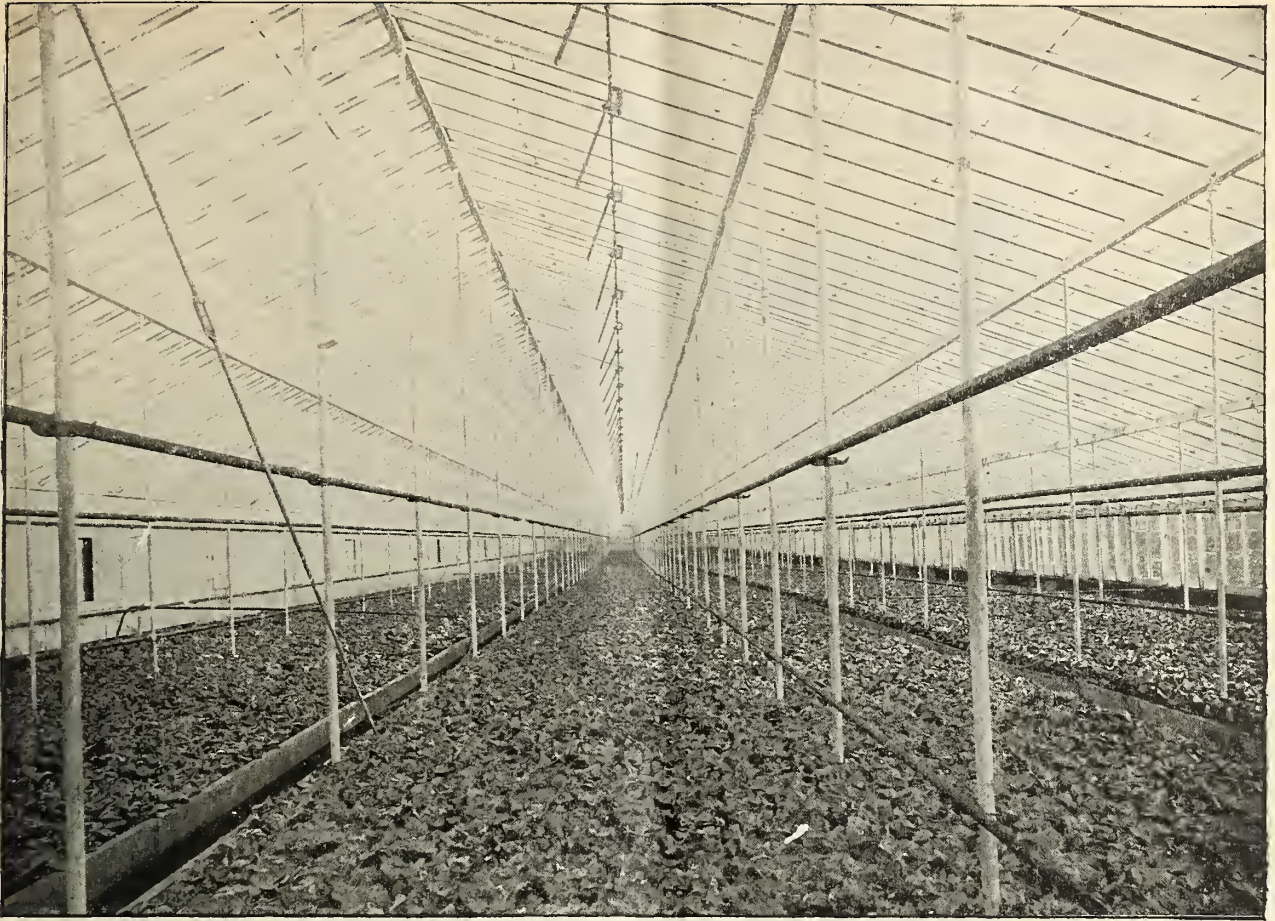
The above photograph was taken in November, when the lettuce was all headed and ready for market. The house is four hundred (400) feet long, and fifty-two (52) feet wide, and contains twenty thousand eight hundred (20,800) square feet, which is nearly one-half acre under the one roof. We grow and mature over thirty-six thousand (36,000) heads of Lettuce in this house at one time. This house is shown in illustration on page 4, being the one in the distance where the electric lights are.
