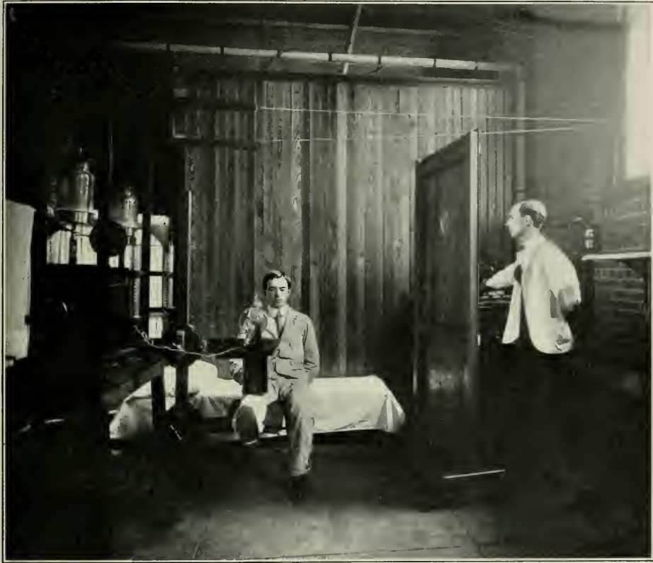
FIG. 208.—Shows how tube-stand table is used when antero-posterior view of knee is desired. Patient is in chair, and leg is placed on adjustable table, as described under compression cylinder. (Original.) The operator may be observed behind the lead screen in which a hole 4 inches in diameter is cut. This hole is covered with lead glass \frac{1}{4} inch thick.
