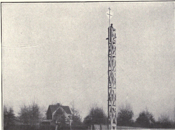
STRUCTURE FOR ELEVATING SIGNAL LAMP OVER TRIANGULATION STATION USED AS MARK.
