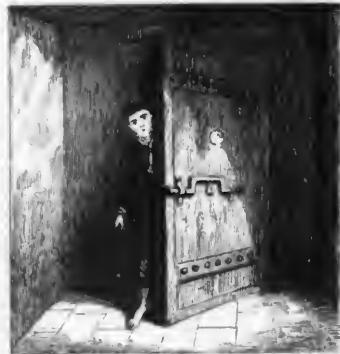
A door between the Red Room & the Chapel
