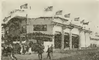
The Derby Racer of Ocean Park It is built with KELLASTONE
