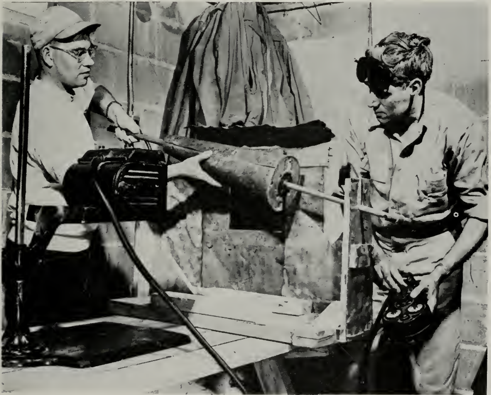
Fig. 4.—An X-ray head and fluoroscopic screen used at the Havana laboratory of the Illinois Natural History Survey to determine the incidence of ingested lead shot in wild waterfowl trapped alive as well as in dead and moribund birds picked up in the field. Each bird was placed in the cone, which was rotated in front of the fluoroscopic screen. This procedure presented to view more than one plane of the bird's body and thereby resulted in more precise location of pellets than was possible in a single plane view. (Photograph from the Journal-Star , Peoria, Illinois.)
