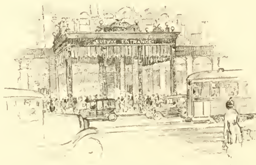
The Stores are connected directly with the Subway
