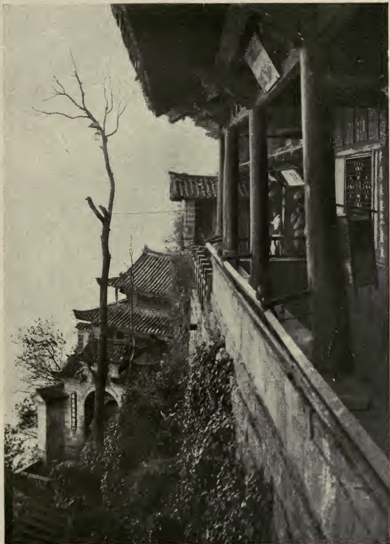
CHINESE ARCHITECTURE ON A STEEP MOUNTAIN SIDE.
