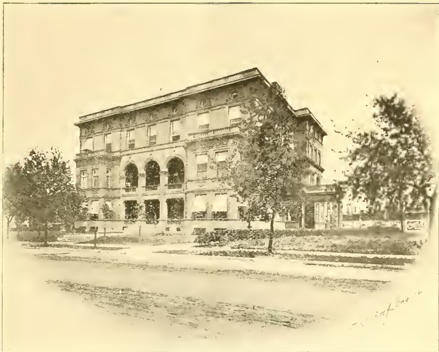
The Columbian Club Building N. W. Corner Lindell and Vandeventer Aves
