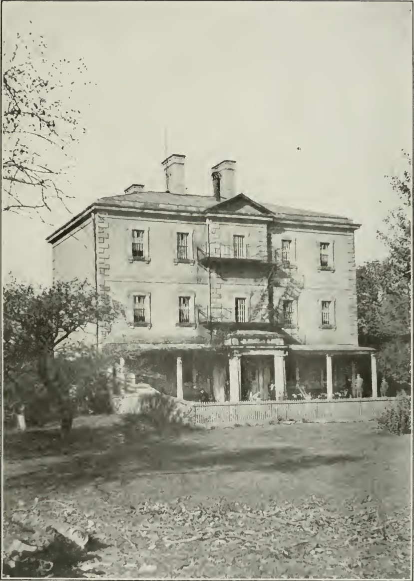
South Cottage, Toronto.
