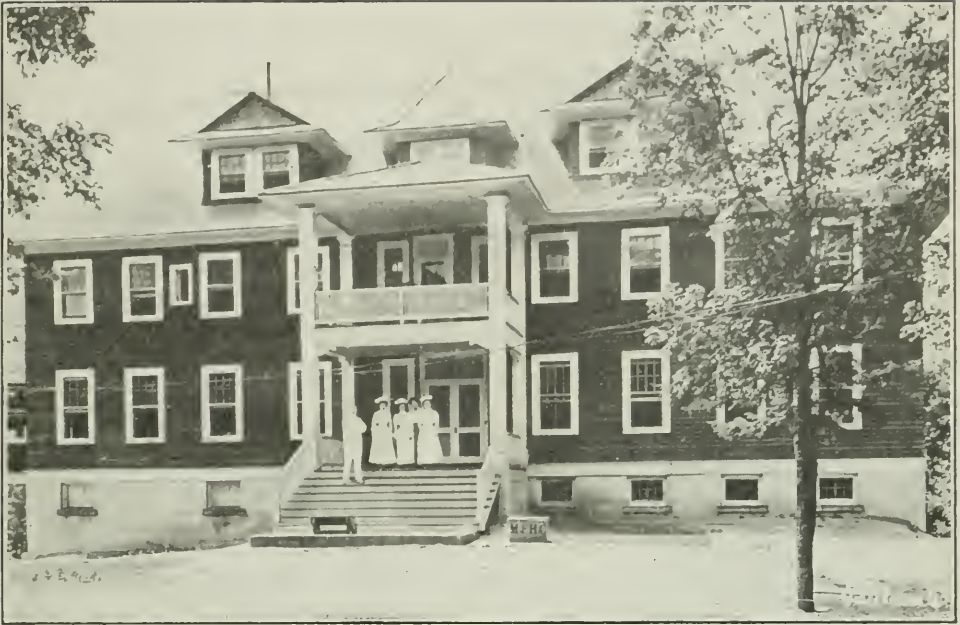
Main Building. Free Hospital for Tuberculosis, Gravenhurst.
