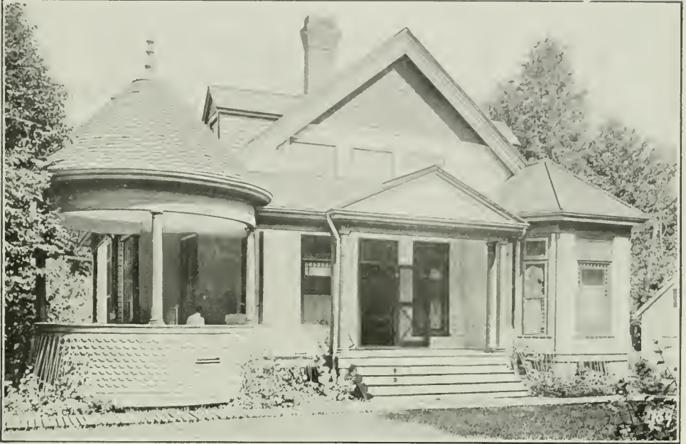
Cottage. Muskoka Cottage Sanatorium.
