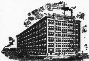
FACTORY 132 ND TO 133 RD ST & BROOK AVE
