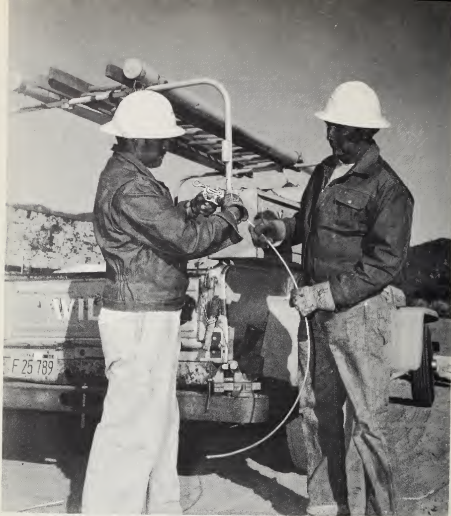
Two mission Indians, Matt Gonzales and Simon Arenas, wiring a hot line clamp.
