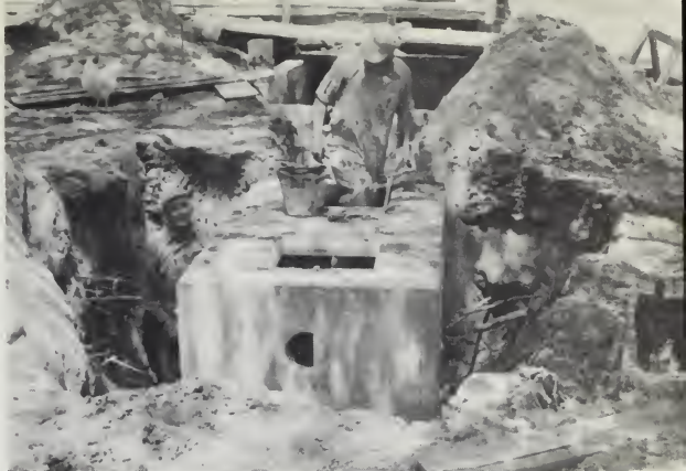
Rosebud Electric News uses photos to explain septic tank installation.
