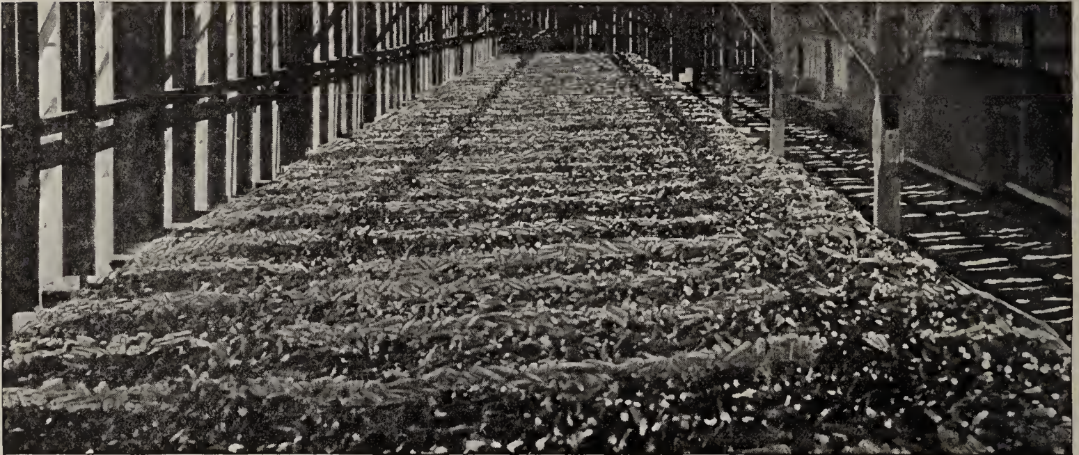
A Corn Drying Shed — Total Capacity 3,000 Bushels
