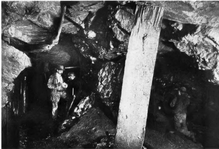
14. HEANE, LOOKING WEST, BLUE HILLS MINE.
