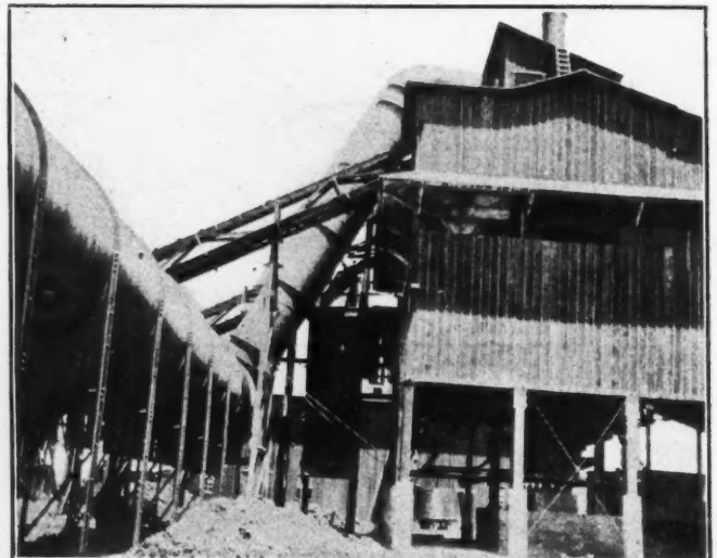
FIG. 8. FURNACE BUILDING AND DUST FLUE
