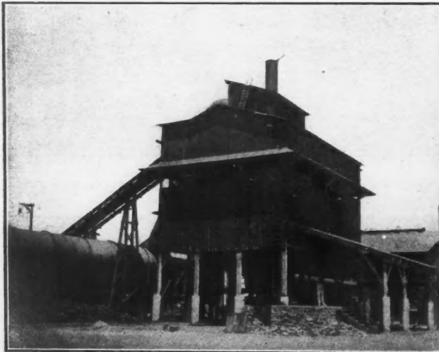
FIG. 7. FURNACE BUILDING FROM SLAG DUMP
