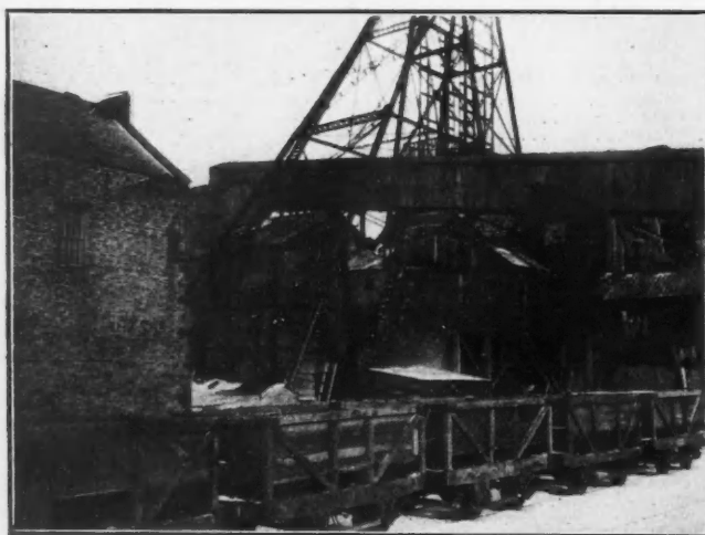
FIG. 3. SHOWING ROBINS CONVEYER DELIVERING SLACK TO WASHERY
