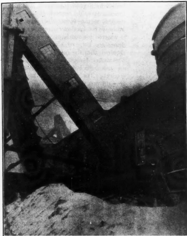
FIG. 5. ELEVATOR FROM WASHER TO TOWER, AND PIPES CARRYING SEA WATER FOR SLATE FLUSHING
