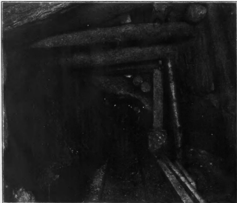
STOPE NO. 17 AFTER CLEARING AWAY THE DEBRIS
