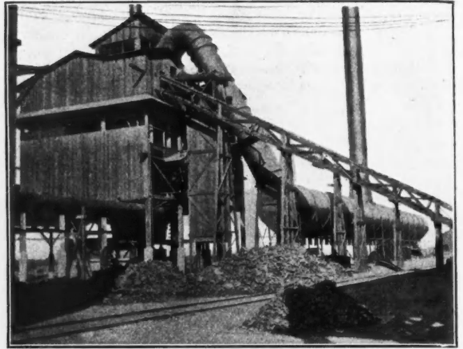
FIG. 6. GENERAL ARRANGEMENT, NO. 1 COPPER FURNACE
