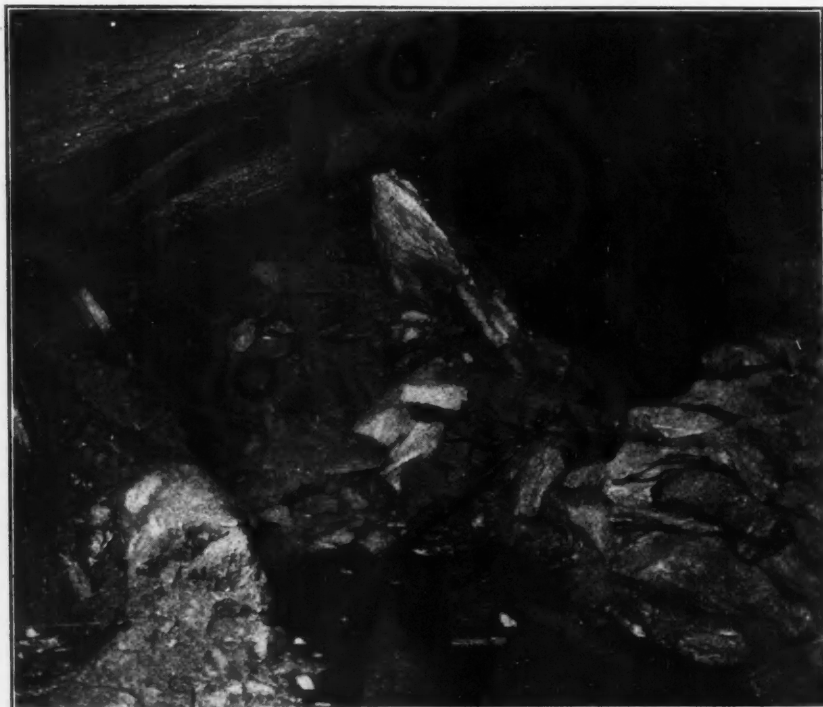
CONDITION OF STOPE NO. 17 AFTER THE SQUEEZE
