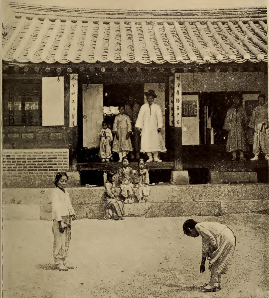
A YANGBAN'S RESIDENCE—ENTRANCE.
