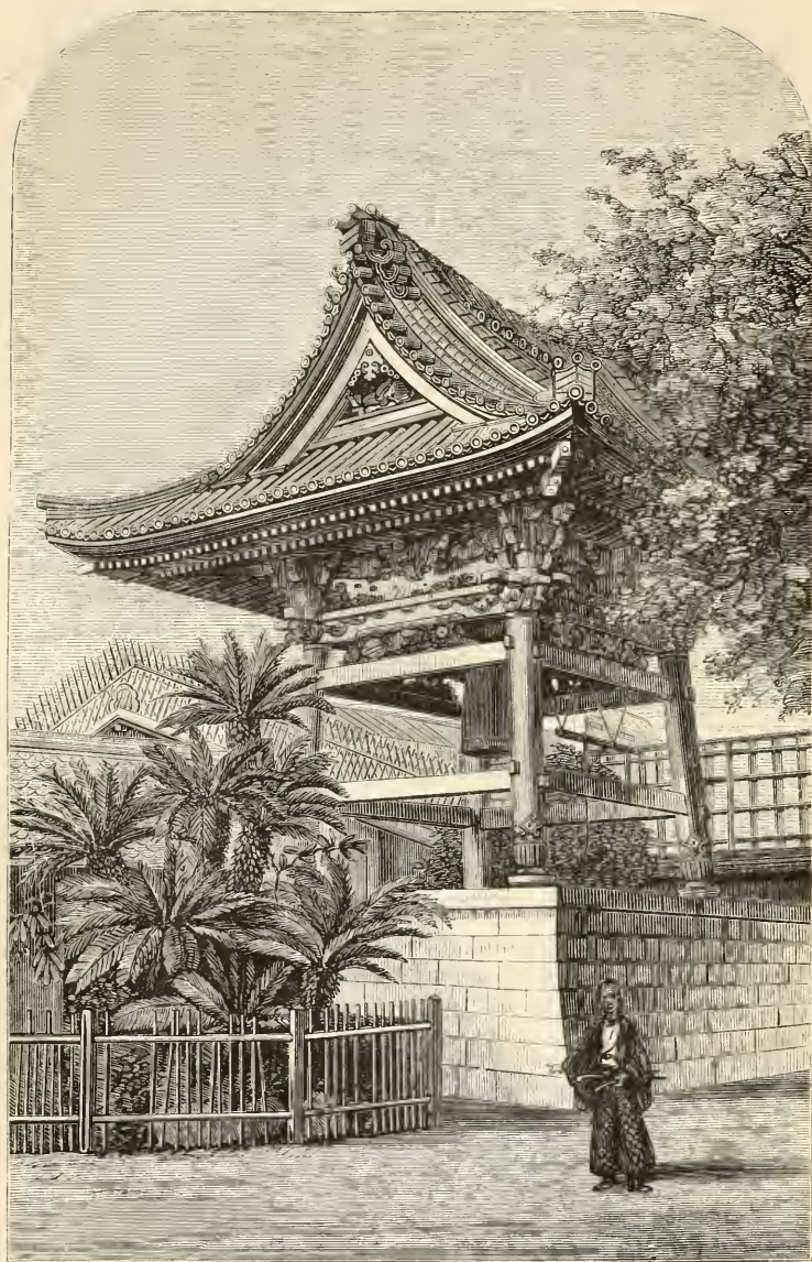
BELFRY IN COURT-YARD OF TEMPLE.
