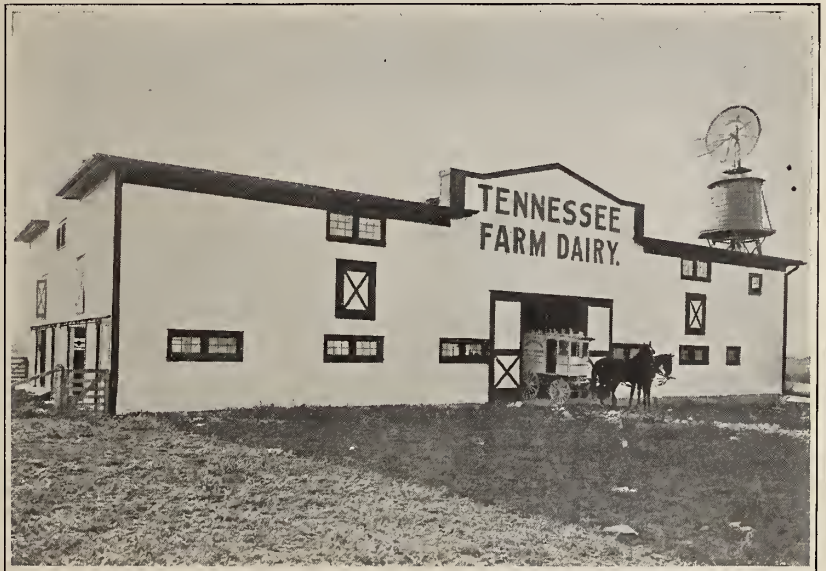
EXTERIOR VIEW OF DAIRY BARN
