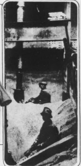
THIS IS THE WAY IT'S DONE —Did you think they had to shovel out wheat carried in bulk in the holds of ships? They don't. This U. S. Shipping Board vessel at Naples, Italy, is unloading its grain cargo by means of a rubber hose operated by suction.
