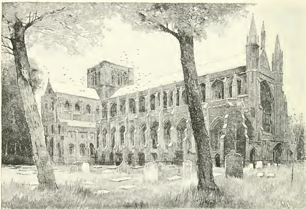
THE NAVE AND TRANSEPT, FROM THE NORTHWEST.
