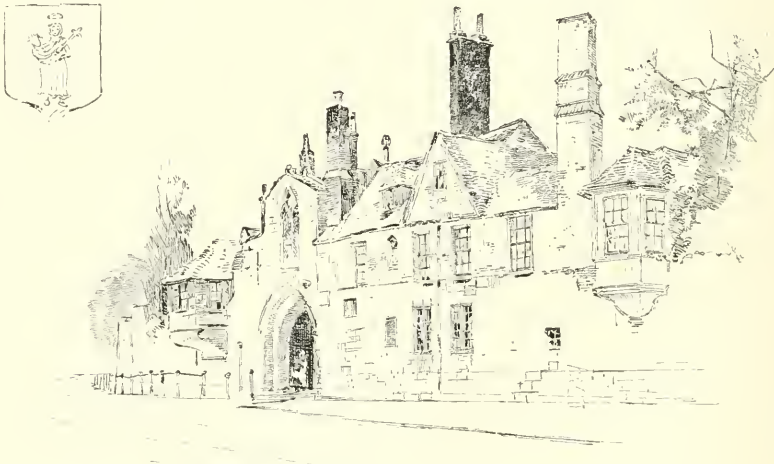
NORTHEAST GATEWAY TO THE CLOSE.
