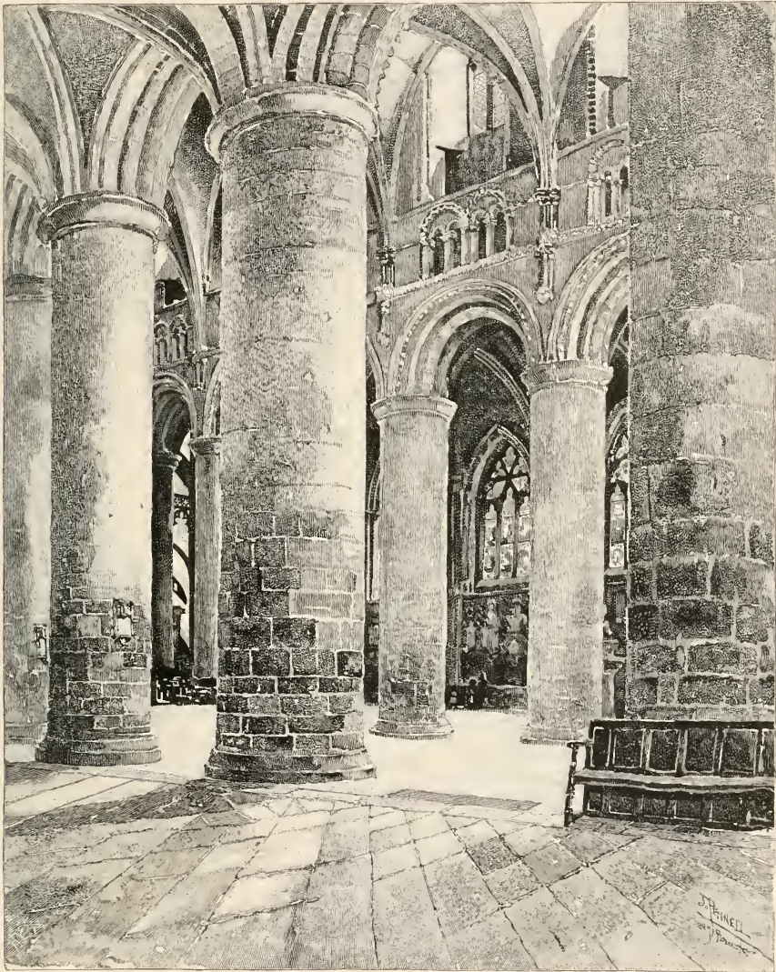
THE NAVE, FROM THE NORTH AISLE.
