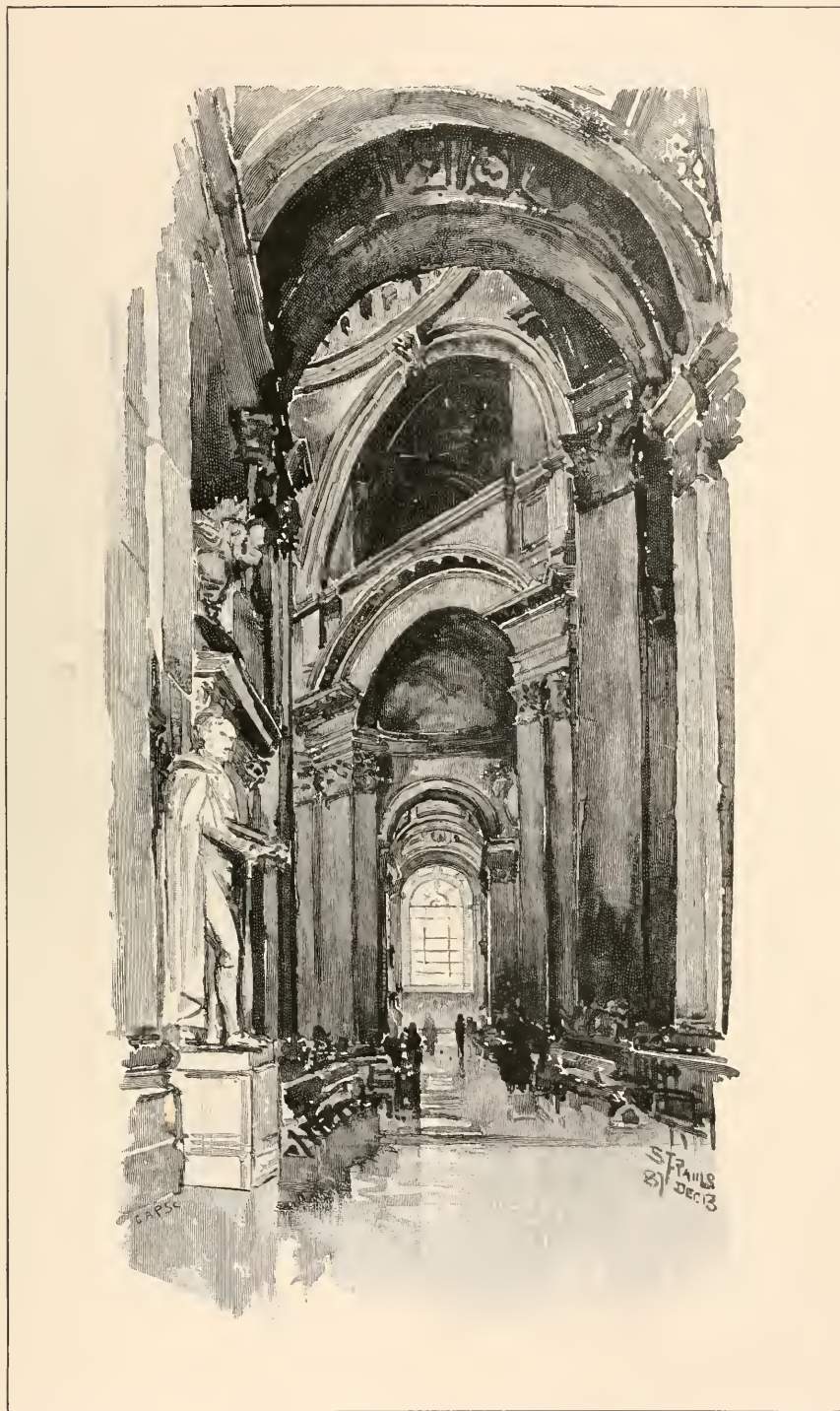
THE WESTERN AISLE OF TRANSEPT
